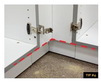
16. Filler should be flush with the front of cabinet body & bottom of cabinet. Secure in place with fastener screws in the previously marked areas.
