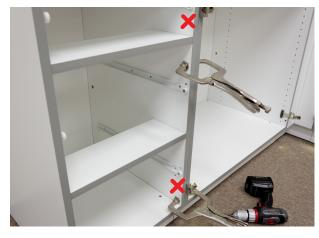
18. Clamp each cabinet's sides together on the top and bottom. Select a system hole near the top and bottom of each cabinet to use for joining.
