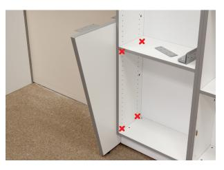
3. Once support panel is positioned and the top is level with base cabinets, secure in place with screws using the system holes.
