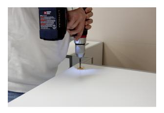
6. Drill pilot holes in the marked spots on the top of each base cabinet.
