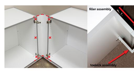
15. Test fit the filler assembly making sure that it is flush with the top and bottom of the adjacent base cabinets. Select three (3) spots to drill pilot holes for securing filler assembly. The top interior shot illustrates how the filler nests in front of the toekick assembly to create an overlap.
