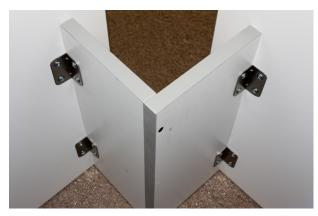
13. Attach the toekick assembly to the outside of each adjacent cabinet as this view from behind shows.
