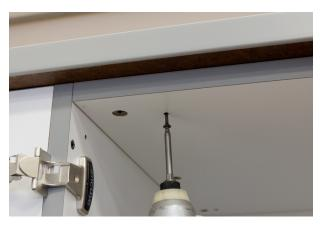
8. After scribe cutting the work surfaces, place and fasten them down with screws from underneath using the pilot holes.
