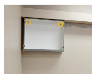
7. Once the cabinet is positioned according to plans, locate the two access holes to begin leveling the cabinet.
