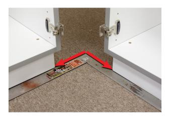
9. Base cabinet corner fillers consist of a lower toekick and an upper filler assembly. First measure and cut the toekick assembly to width.
