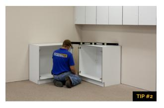
8. Place the next cabinet according to plans and raise it so that its top is level with the first cabinet.
