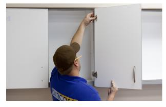
20. Reattach the door fronts to each cabinet by pressing the hinge into the door mount. You should hear a click when it seats properly.
