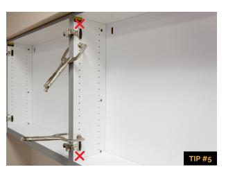
12. Clamp each cabinet's sides together on the top and bottom. Select a system hole near the top and bottom of each cabinet to use for joining.
