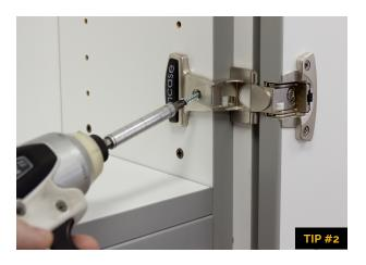
6. After the door is aligned properly, lock each hinge in place with one (1) set screw. Product warranty is void without proper use of set screws.
