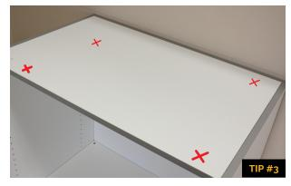
5. Mark drill hole positions on the top of each cabinet where you intend to fasten the work surface down.
