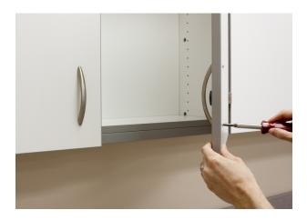
8. The pulls are installed on the inside of each cabinet to protect them during shipping. Take a moment to remove all pulls and install them facing outward.
