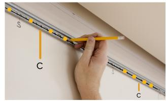
2. Place mounting rail so horizontal line intersects center holes. Mark two (2) holes to drill within 6" of every cabinet side (c).
