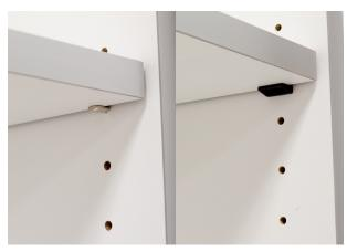
2. Use the metal shelf pins for storage and base cabinet shelving and the black clips for overhead cabinets.
