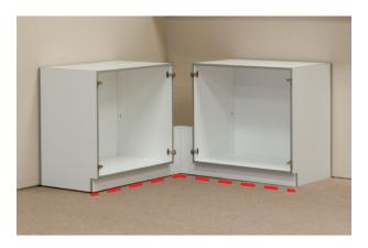
12. Test fit the filler making sure the toekick assembly is flush with the adjacent cabinets' toekicks and flush with the bottom.
