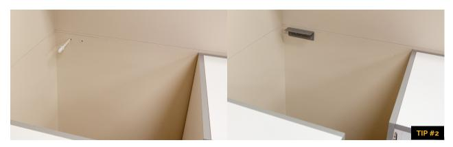
4. Some situations may require additional support in corner applications. Here, an angle bracket is used with togglers and bolts. Drill marked holes with a 1/2" drill bit. Be mindful of services (plumbing, electrical, etc.) in the wall before drilling.
