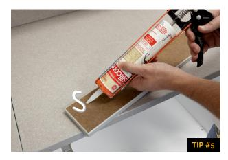
10. Scribe cut backsplashes and sidesplashes to fit. Apply caulk to the back and clamp in place until dry.
