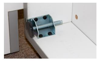
4. Adjust levelers so they are not extended. This first cabinet on the high point needs to sit as close to the ground as possible.
