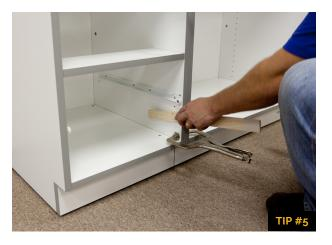
19. Using a 1/4" drill bit, ream one system hole on the top and one on the bottom of the side panels for connecting bolts.
