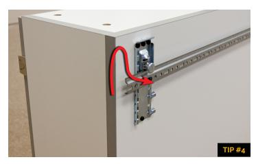
6. Hang the first cabinet on the mounting rail. The circular discs on the brackets must be seated over the lip of the rail.
