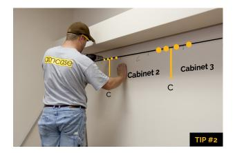
3. Remove the mounting rail and drill marked holes with a 1/2" drill bit. Be mindful of services (plumbing, electrical, etc.) in the wall before drilling.
