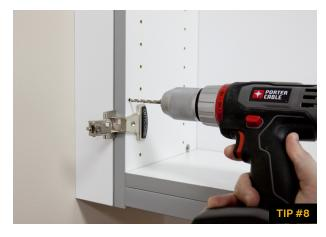
18. Select two (2) or three (3) spots to drill pilot holes for securing filler panel. Filler should be flush with the front of cabinet body & bottom of cabinet.
