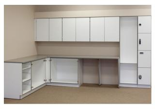
7. Place the work surfaces in place, and scribe cut to fit. Use a jig saw or belt sander as needed to fit the cut edge to an uneven wall.
