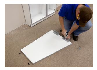
1. Review plans and assemble support panels for work surfaces. Thread levelers into the bottom panel inserts as required.
